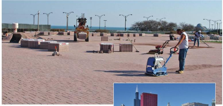
ABOVE: A compactor "locked" the pavers into the bedding aggregate, with a minimal 7-millimeter joint between the pavers. An open-graded crushed granite joint material matching the 'Coral Gem' color was selected to further minimize any visible patterning. PHOTOS: UNILOCK
